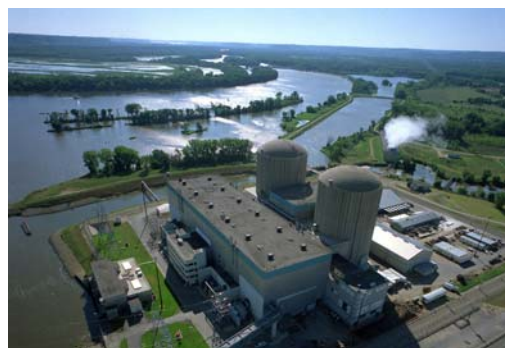
Thermoelectric Power Plant
